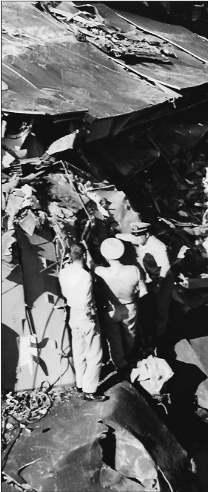
Port side damage inspected on 8 May 1964
